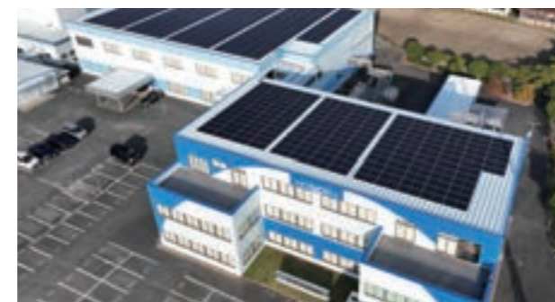
Hosiden Kyushu (Started operation in February 2023)
