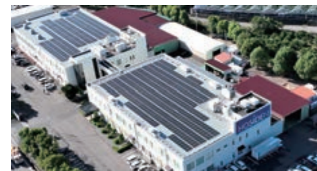
Hosiden Wakayama (Started operation in November 2022)
