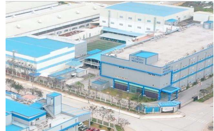
Hosiden Vietnam (Bac Ninh Province) (Image of new building 1,2,3)
