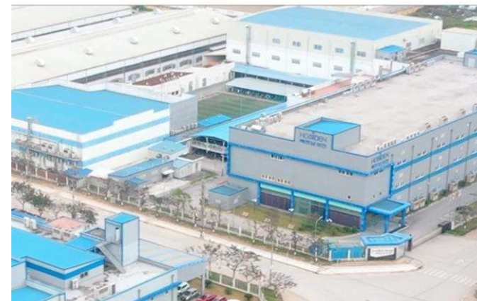
Hosiden Vietnam (Bac Ninh Province) (Image of new building 1,2,3)
