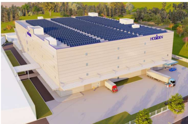
Hosiden Vietnam (Bac Ninh Province) (Image of new building 8)
