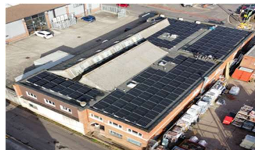
Hosiden Besson 1st phase (United Kingdom)
